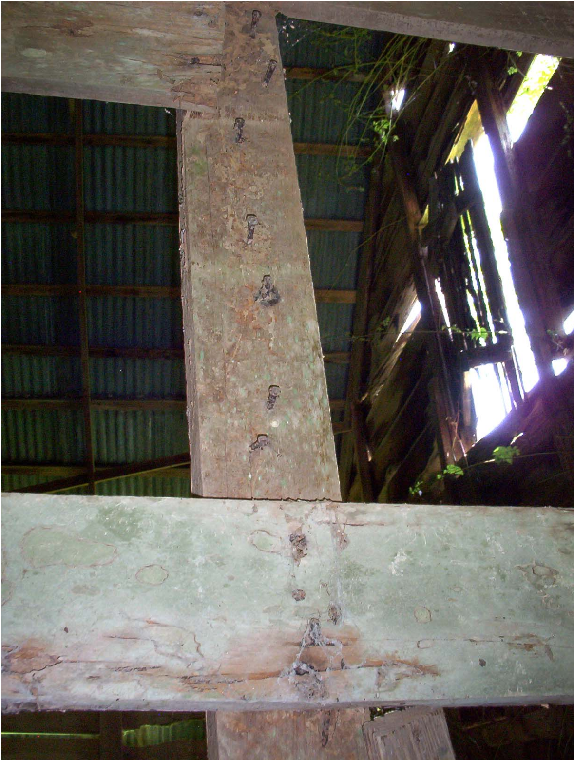
Figure 5.19. Modern machine cut nails hold the planks in place.
