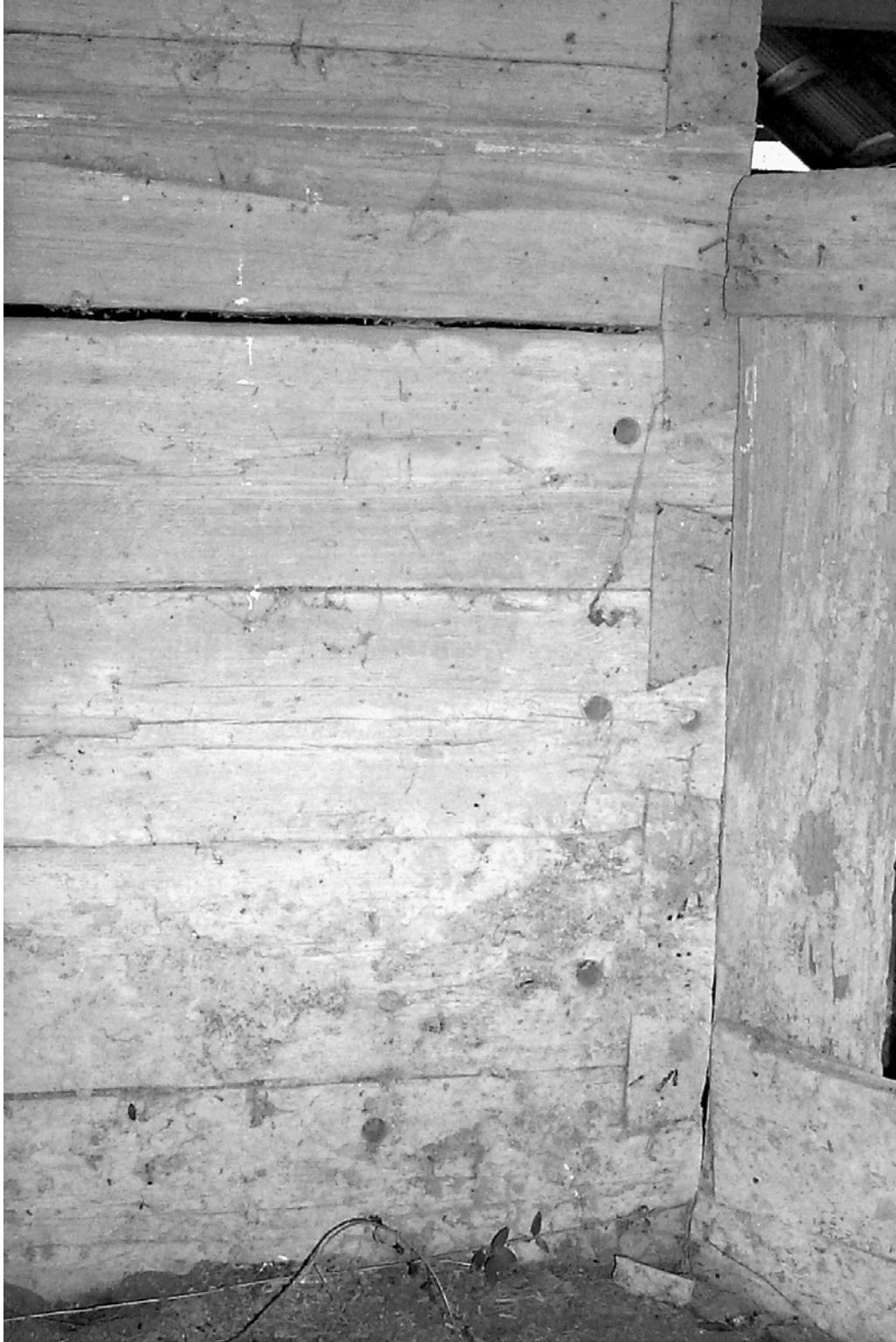
Figure 5.2. Some of the holes in the timbers seen here may have been created to construct timber “rafts,” which were floated from the mill to their final destination.
