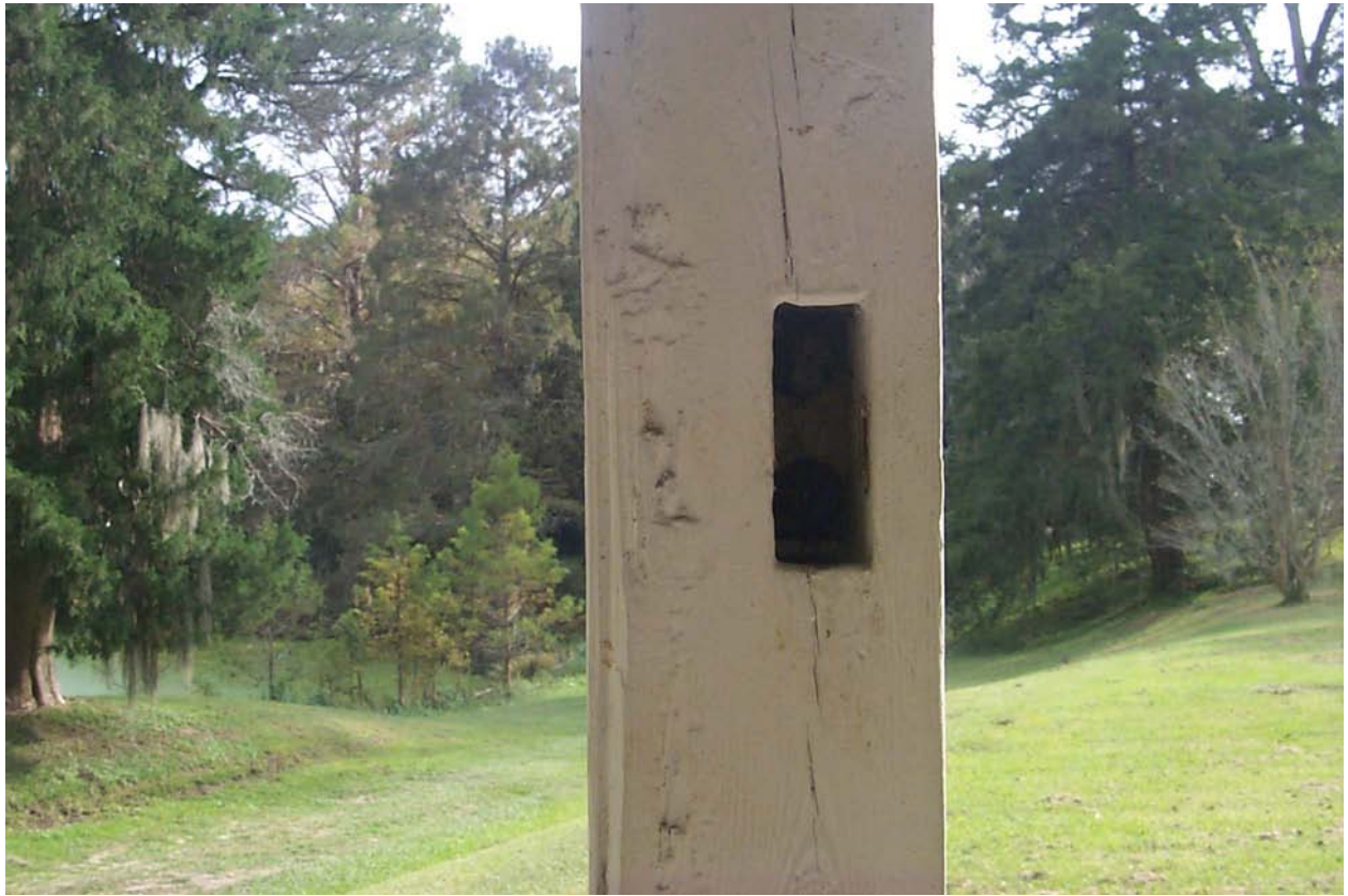
Figure 5.41. Some of the uprights supporting the roof of the Rosedown Milk House were reused from another structure. Note the mortise in this upright.
