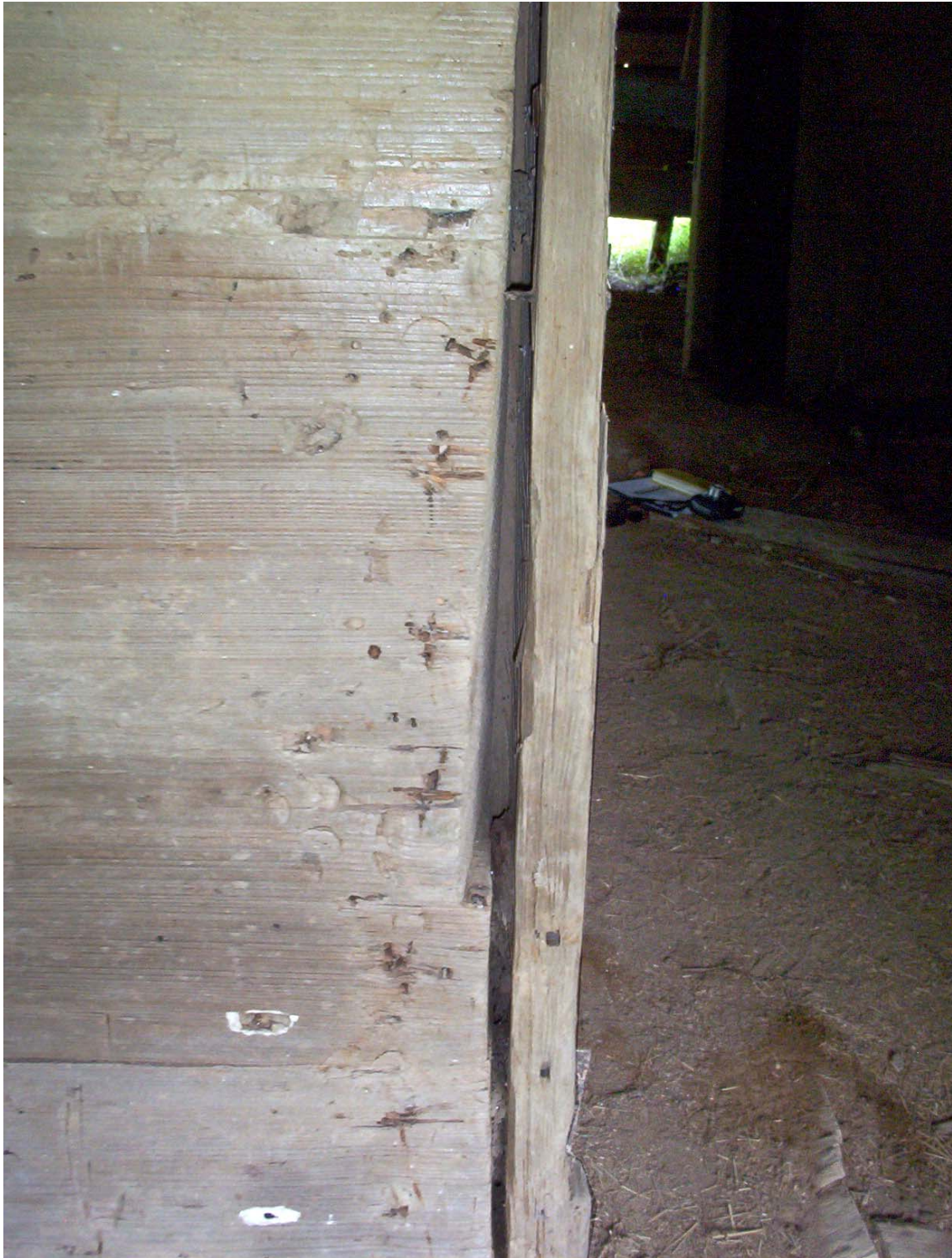
Figure 5.11. The western door opening was added at a later date and was crudely cut into the building.
