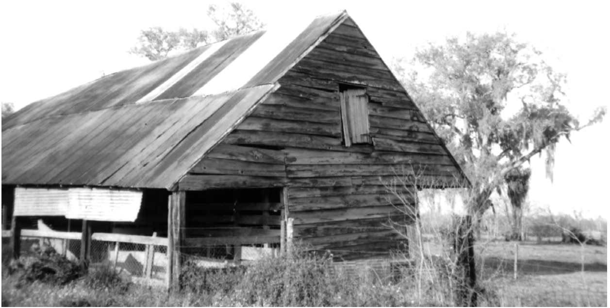
Figure 5.20. Clapboards cover the exterior wall of Room 2.
