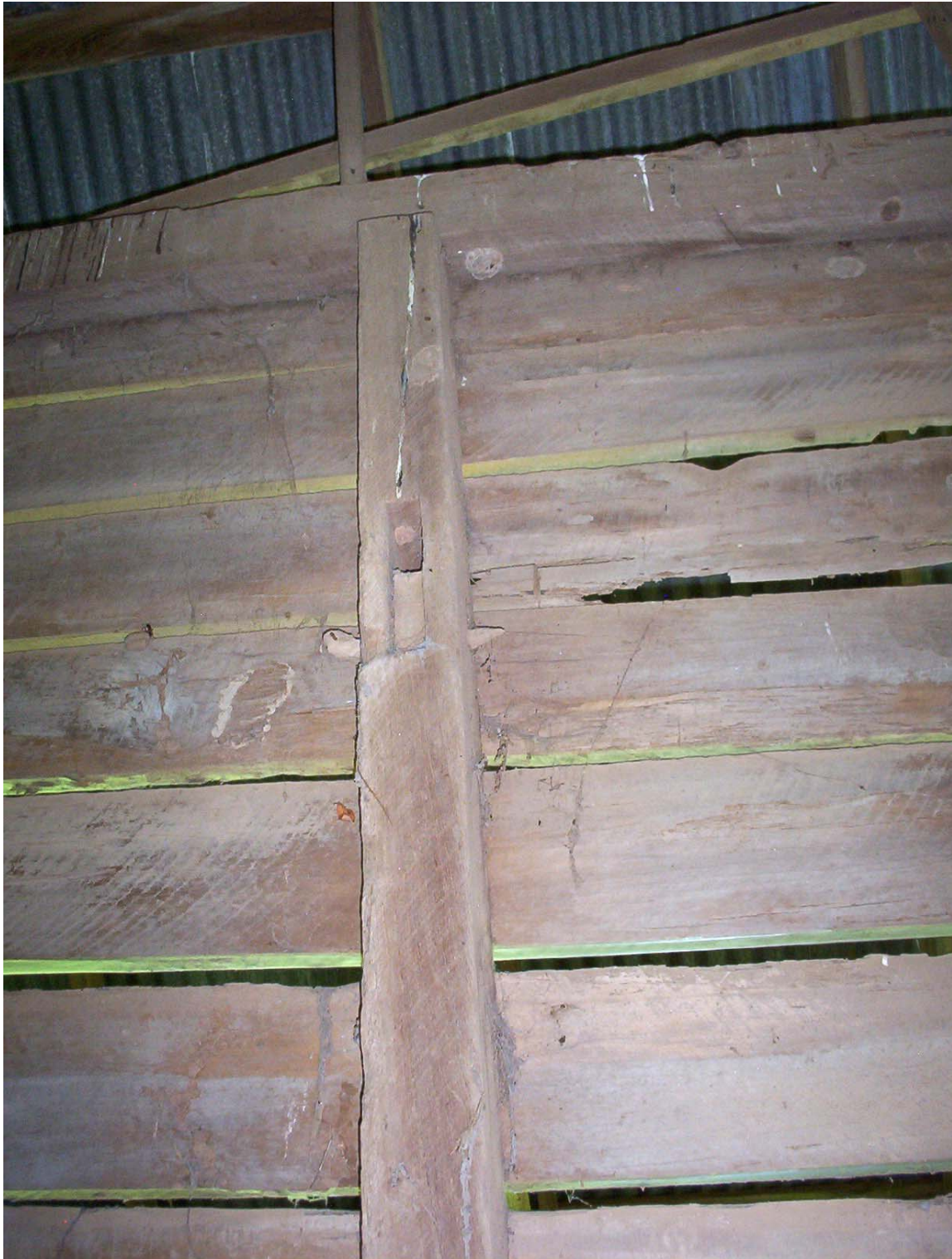
Figure 5.18. The planks that cover Room 2 were circular sawn.
