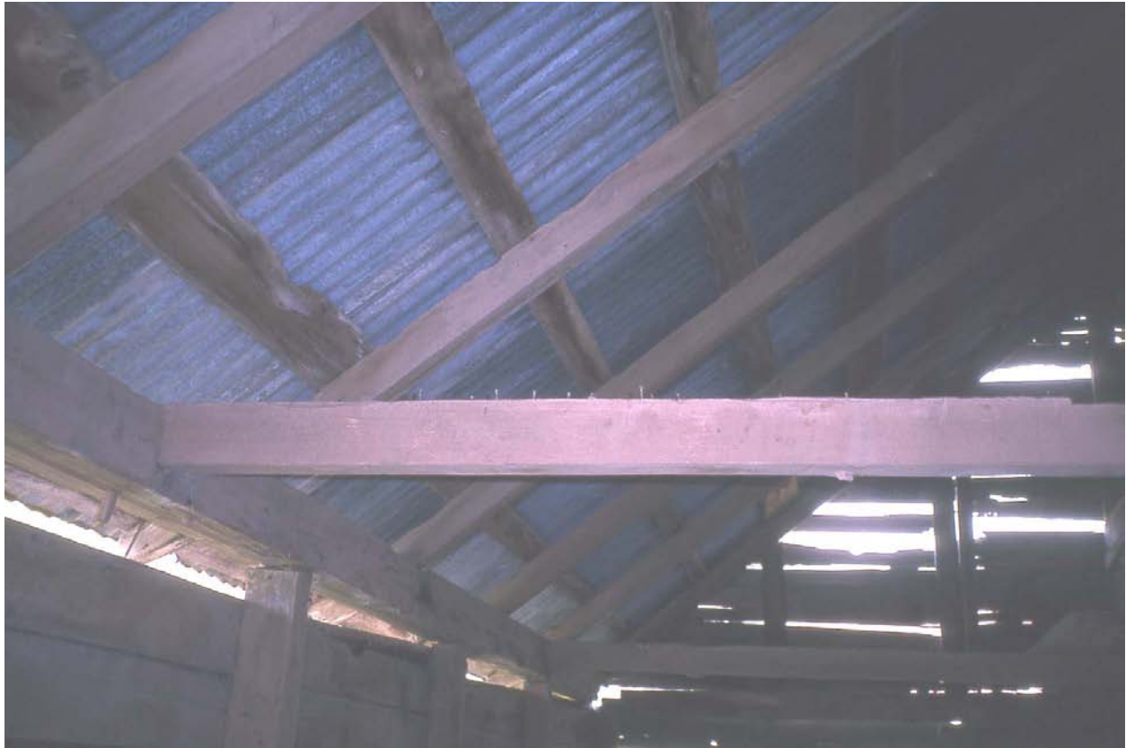
Figure 5.29. The nails shown here on the top of the joist once held wooden planks. This space was probably used for extra storage space.
