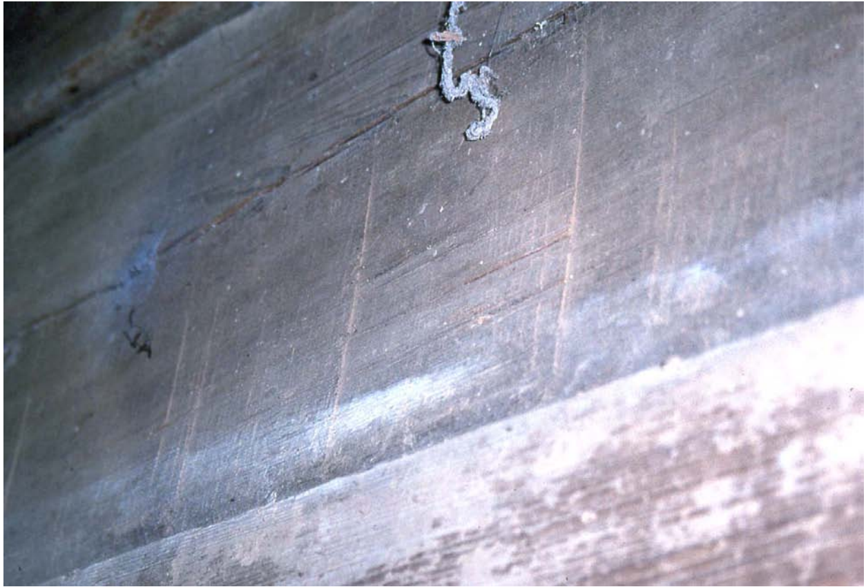
Figure 5.1. Faint sawmarks are visible on the cypress timbers of Room 1.
