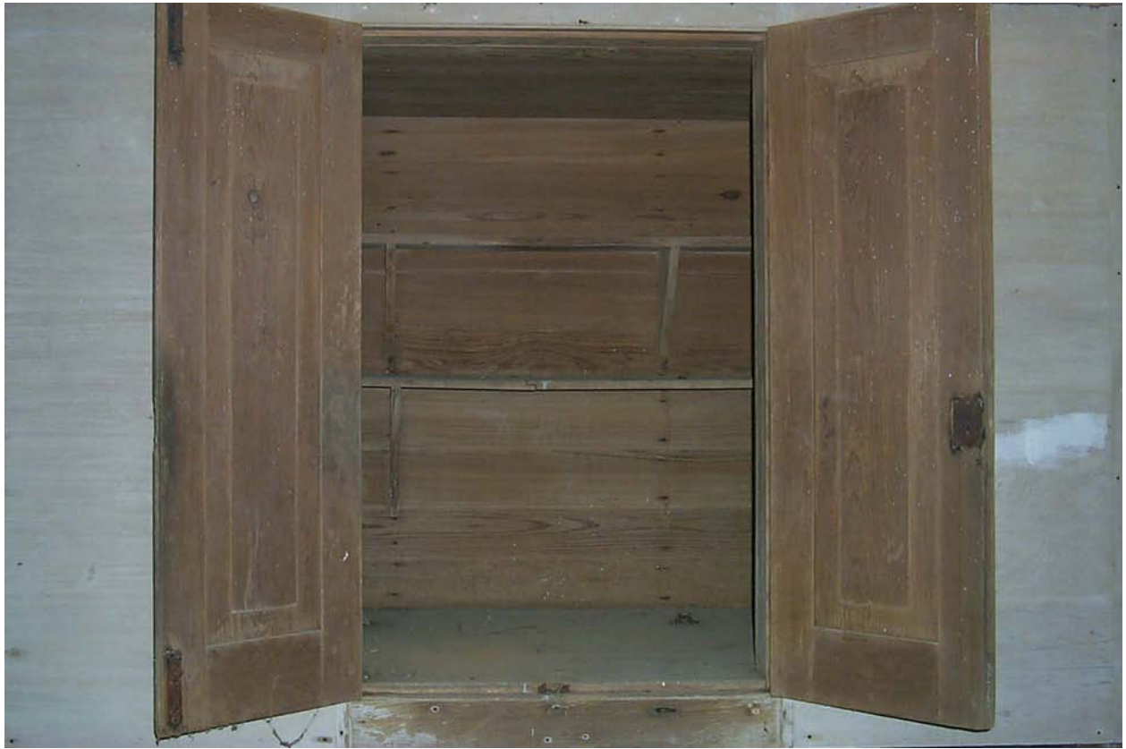
Figure 5.43. This finely made cabinet is located inside the milk house. It was once used to store milk products such as butter and cheese and eggs.
