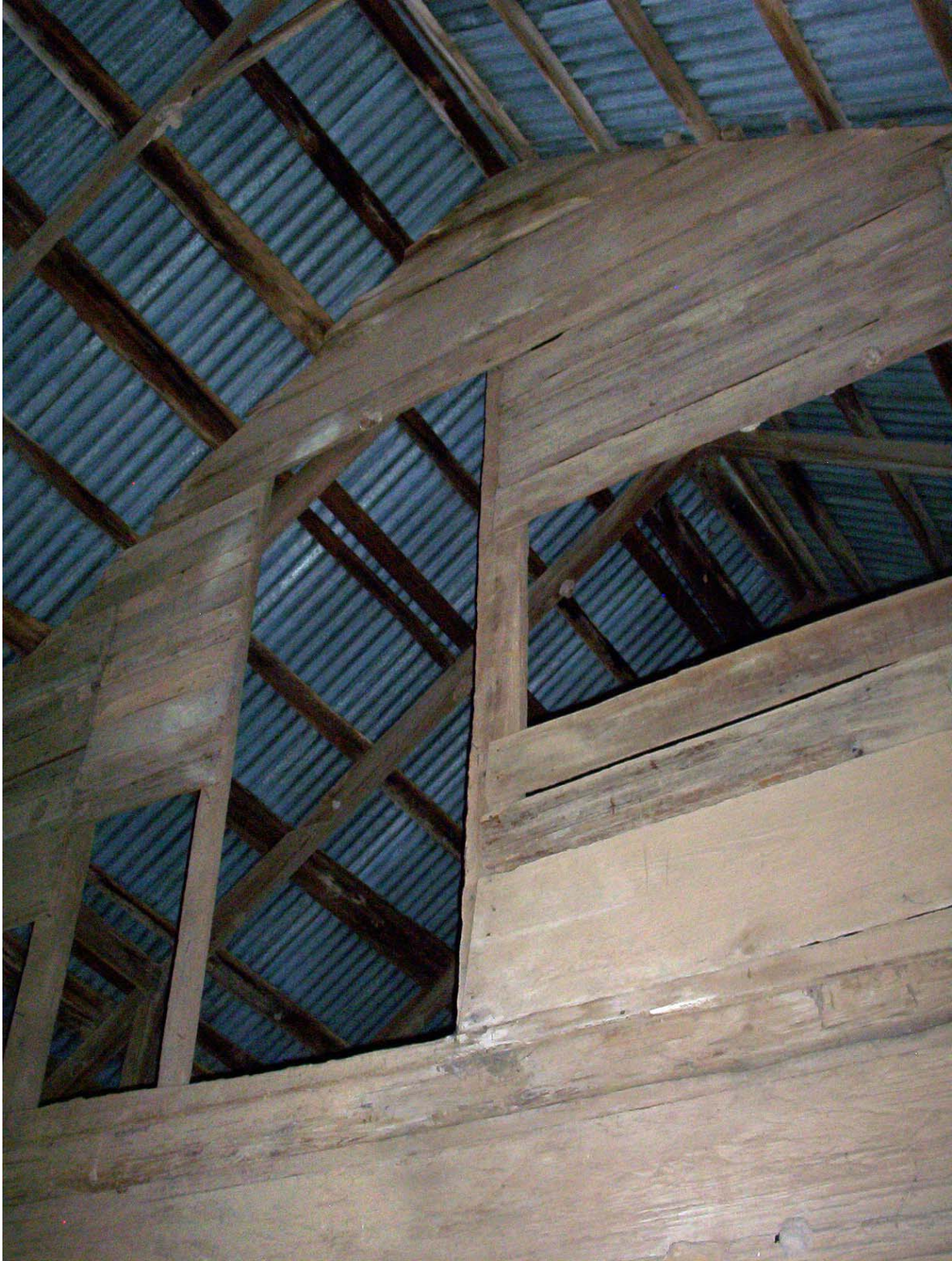
Figure 5.28. This opening may have once held another door to the loft.
