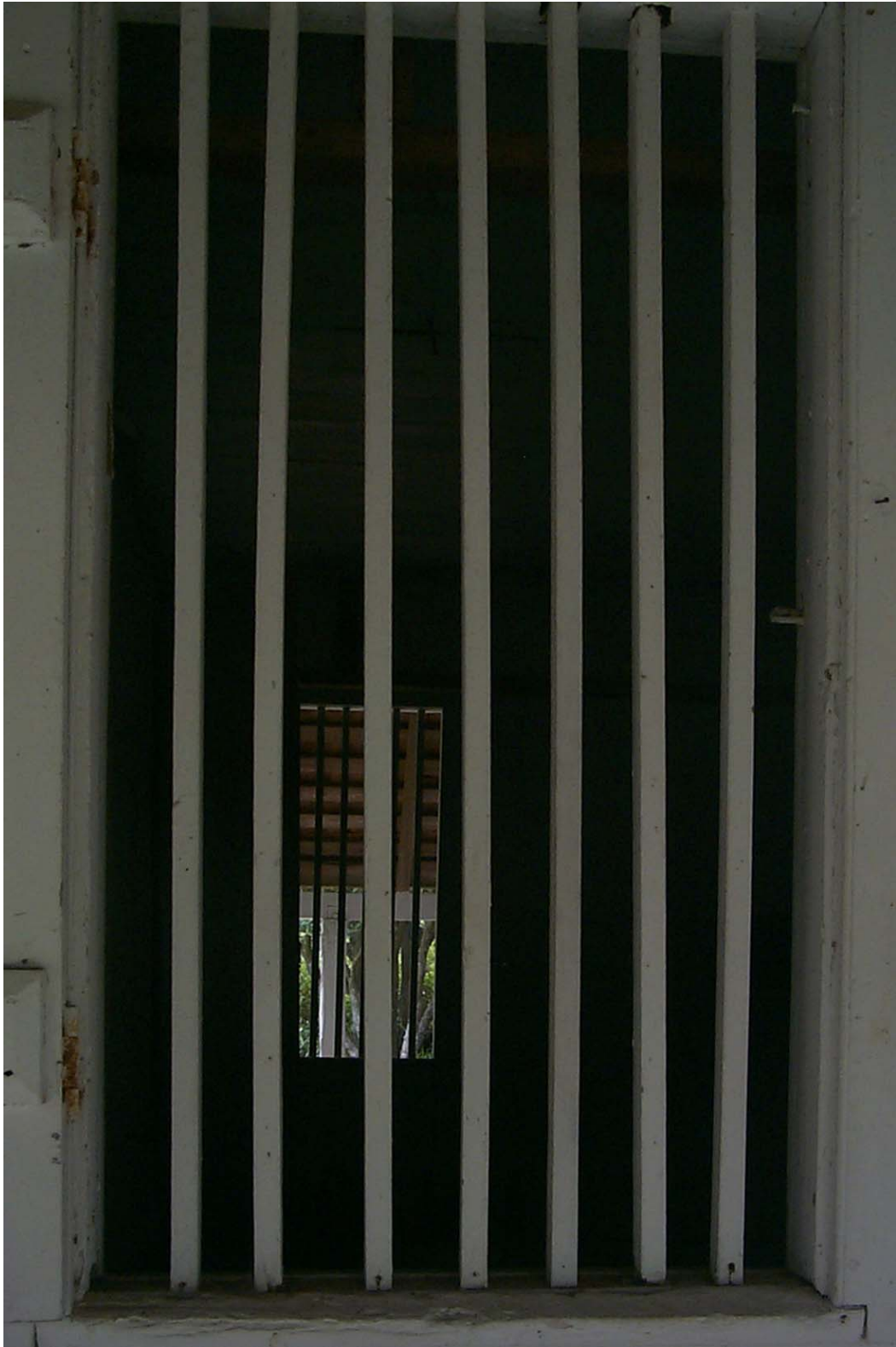
Figure 5.39. Wooden bars keep varmints out but allow the air to circulate.
