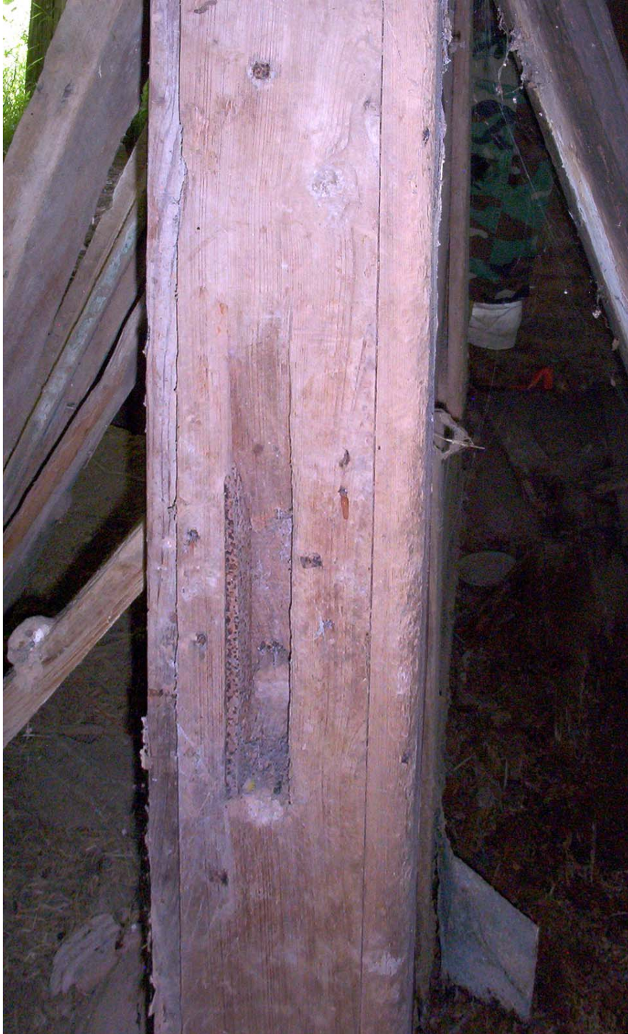
Figure 5.8. Most of the original openings in Room 1 were locked by bar-type latches. Only the notches that the bars slid into remain.
