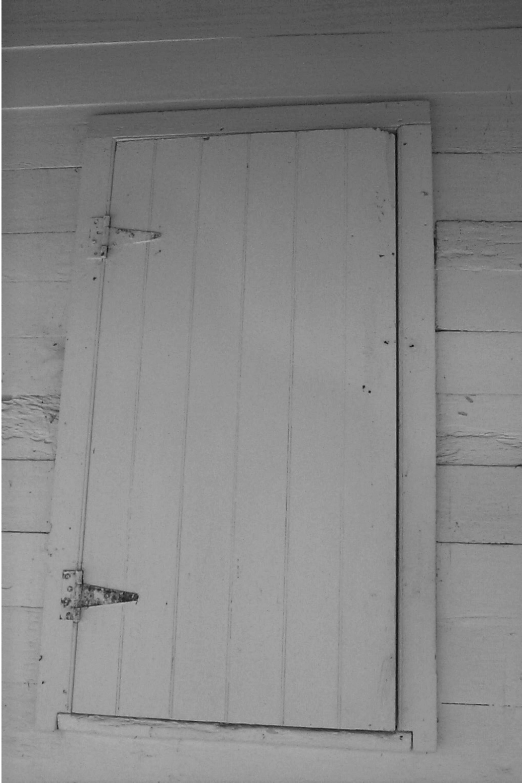
Figure 5.37. The windows and door of the Rosedown Milk House are batten with beaded shutters.
