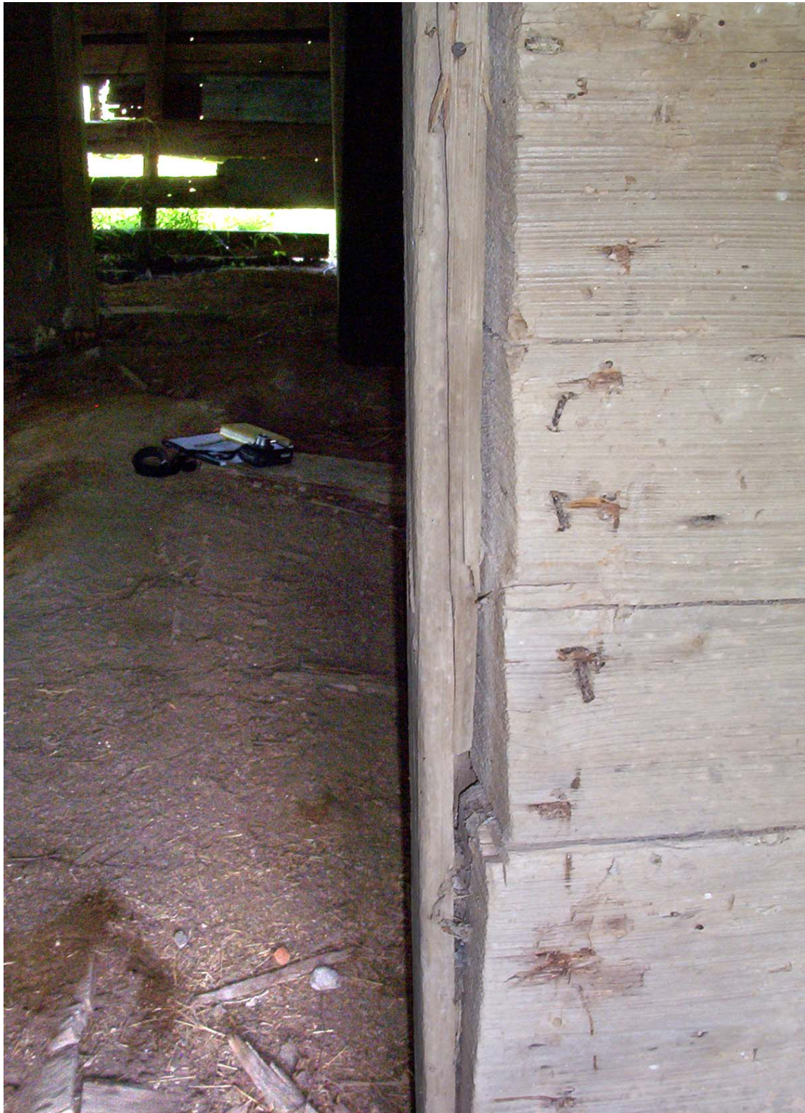
Figure 5.12. Thin boards were scabbed onto the new door opening.
