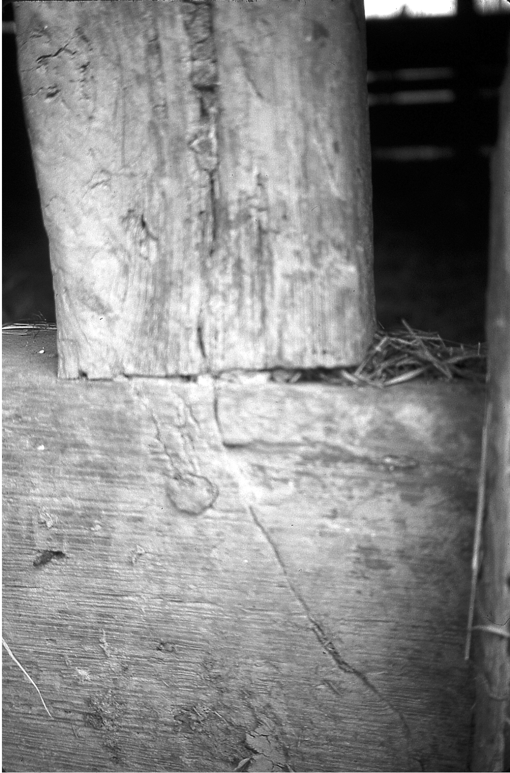
Figure 5.14. Posts are mortised into a sill in Room 2 of the “barn.”
