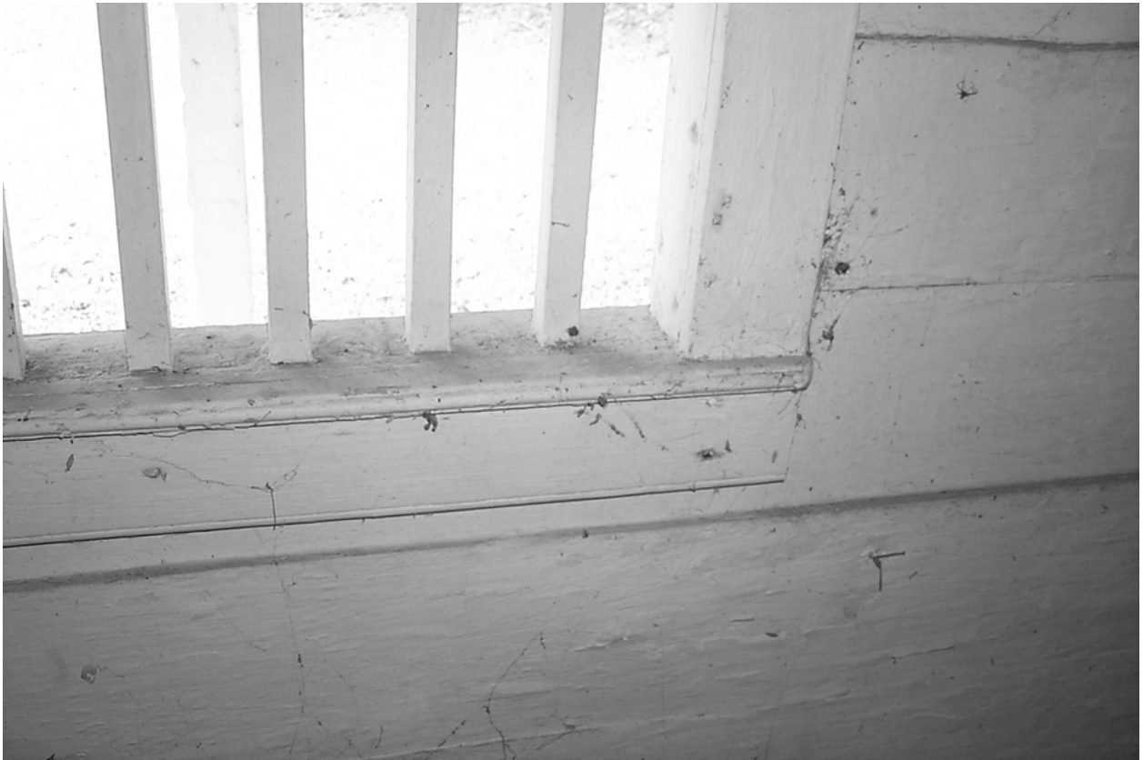
Figure 5.40. Similar to Room 1, the Rosedown Milk House has beaded trim.
