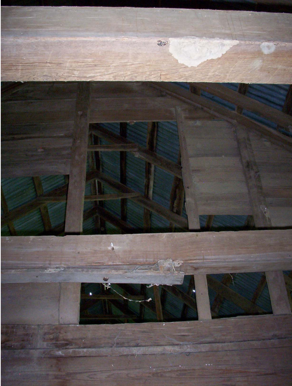
Figure 5.5. Ceiling joists measuring 3.5 by 5 inches are still present in Room 1.
