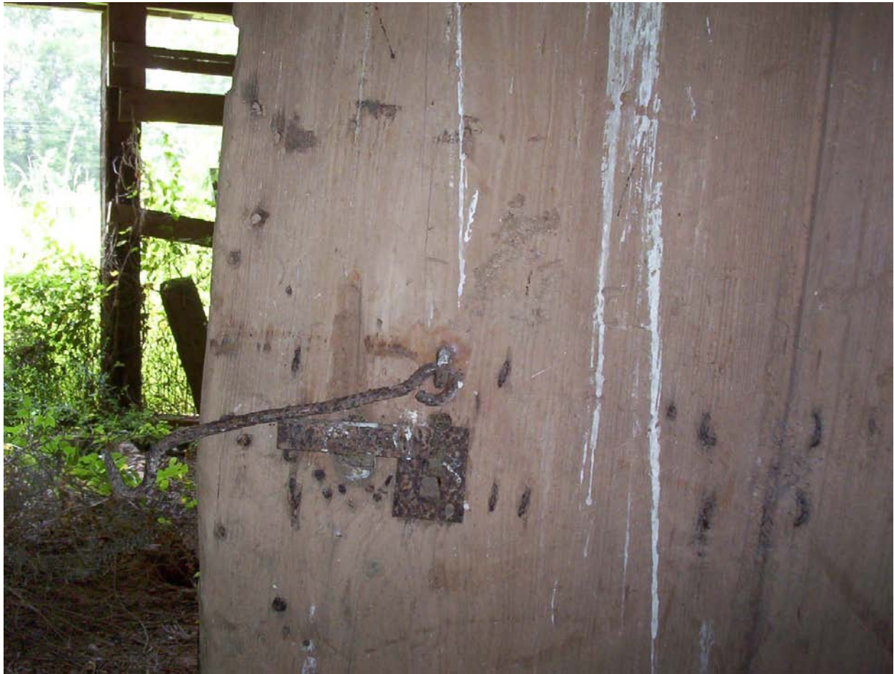
Figure 5.10. All that remains of the mortise-type lock of the southern door of the building is the keyhole.
