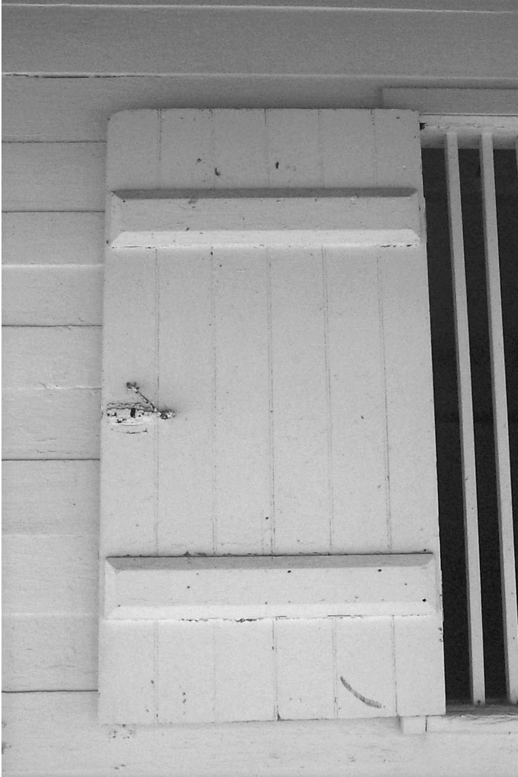
Figure 5.38. Metal latches lock the windows from the inside of the building.
